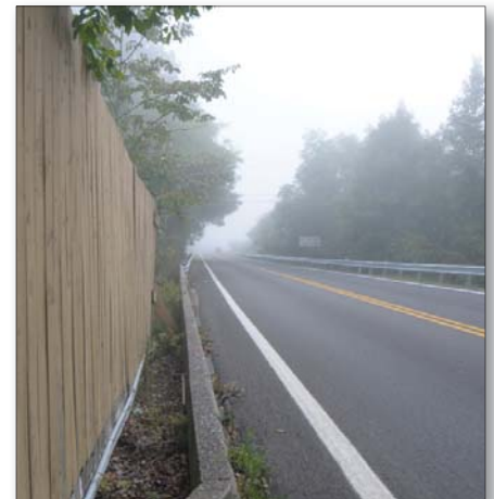
U.S. Route 11 as it crosses over Natural Bridge.
