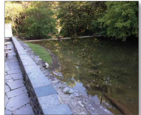
Sedimentation and storm debris have collected upstream of one of the property's dams.
